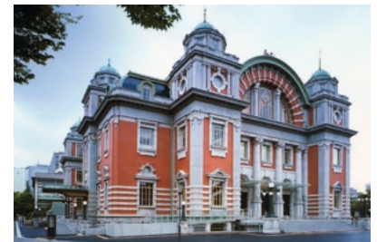
Osaka City Central Public Hall
