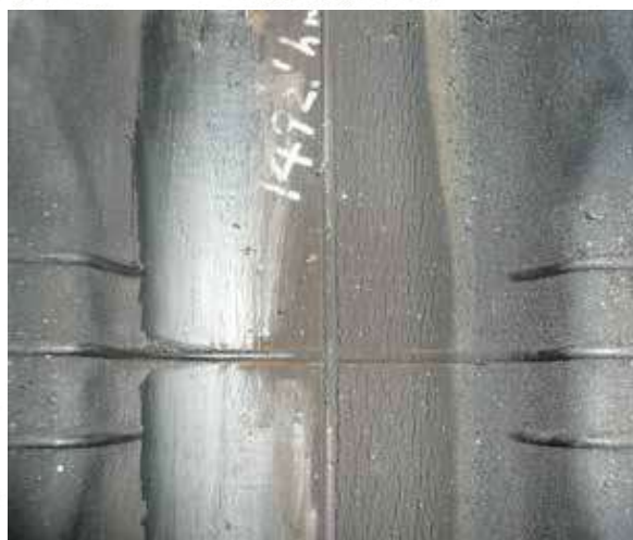
Small ozone cracks
