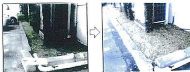
Figure 2. Preventing Weed Growth by Carpeting Open Areas with Wood Chips
