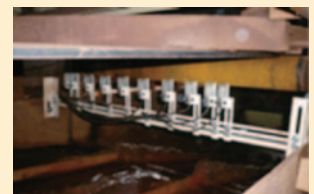
Monitoring system installed on a conveyor belt
