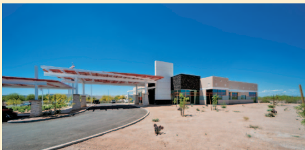
View of Biorubber Process Research Center (under construction)
