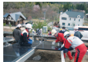
Volunteer activities (solar panel installation work) in Iwaki, Fukushima Prefecture
