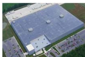
EPDM Roofs (Roofing)
