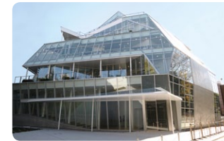
BIG-T Bridgestone Institute of Global Training: This center, which is used by employees from around the world, plays an important role in global conferences and includes facilities for human resources training.
