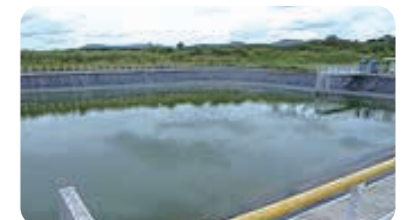
Rainwater collection pond at Bridgestone Carbon Black (Thailand) Co., Ltd. (BSCB)
