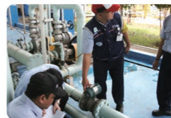
On-site inspection at Bekasi Plant, Indonesia
