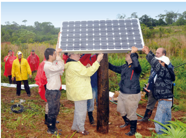
Installation of solar panels
