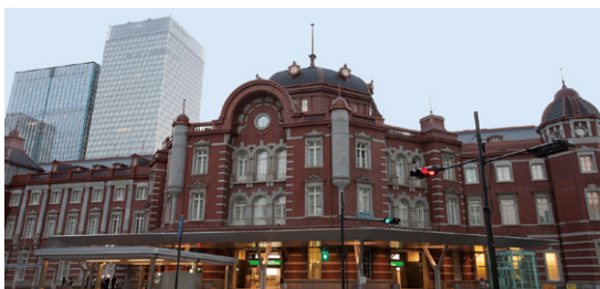
Tokyo Station Marunouchi Building, which adopted Bridgestone elastomeric seismic isolation bearings
