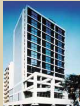
Company's House Company's House Amitei Shin Osaka Design: Shimizu Corporation Construction: Shimizu Corporation
