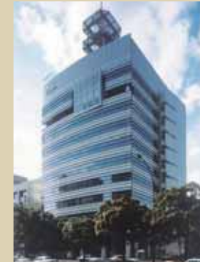
Communication Facility NTT Docomo Shikoku Design: NTT Facilities Construction: Taisei Corporation
